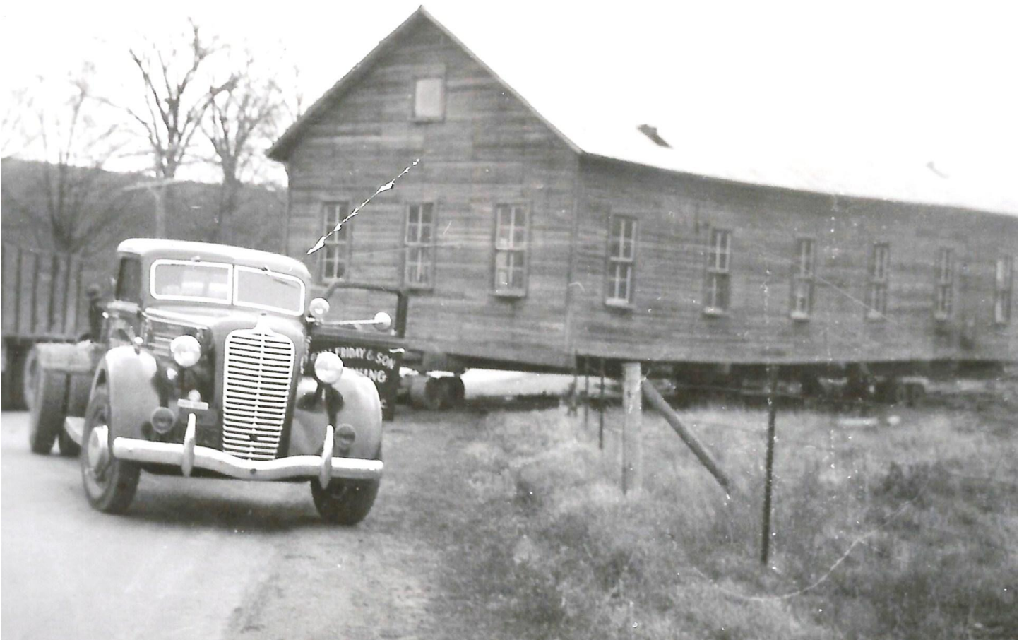
The Spangler Blacksmith shop on the move to its present location in Gillingham. The shop was jacked up on rollers and pulled along Highway 56 by Guy Friday's Trucking Service and placed on a stone foundation where it could be connected to the REA lines. Mary Ann Metz photo.
