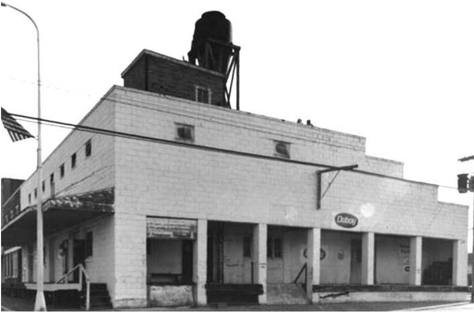
Above: The rebuilt upper mill at 279 West Court Street. Below right: The Good Friday fire of March 25, 1948.
