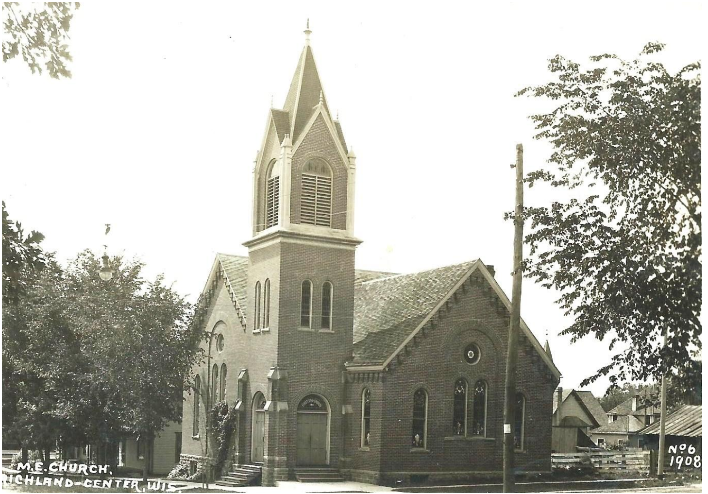
First Methodist Episcopal Church, 258 East Mill Street. Photos from SandHill Marketing collection.
