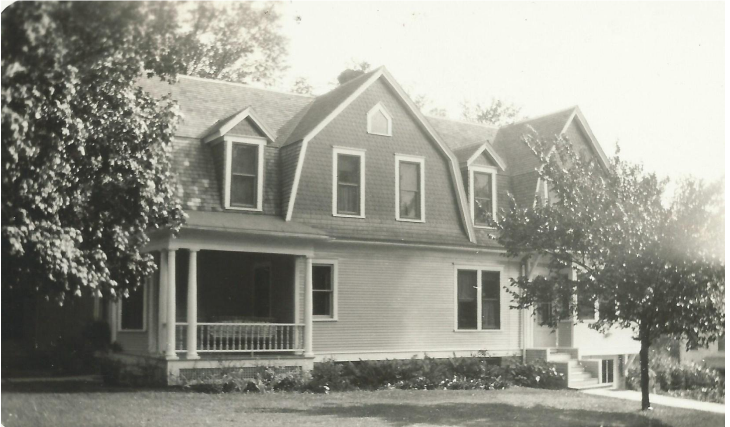
First Street view showing the Smith's 1925 garage addition - Unbehaun photo.
