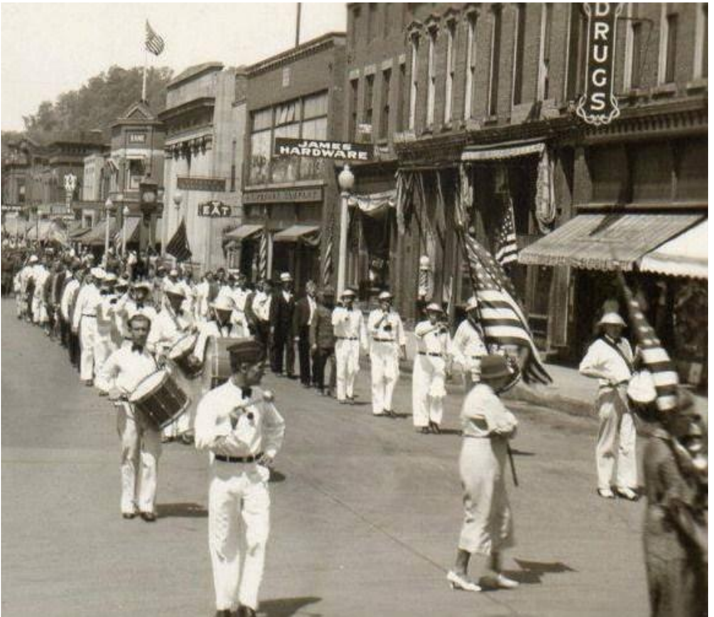
D.G. James Building (adjacent to James Hardware) 172 East Court Street - 1889 - Richland County History Room photo.
